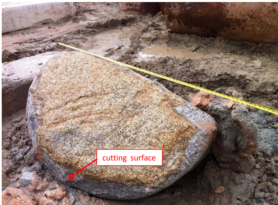
Boulder removal (転石撤去状況)
