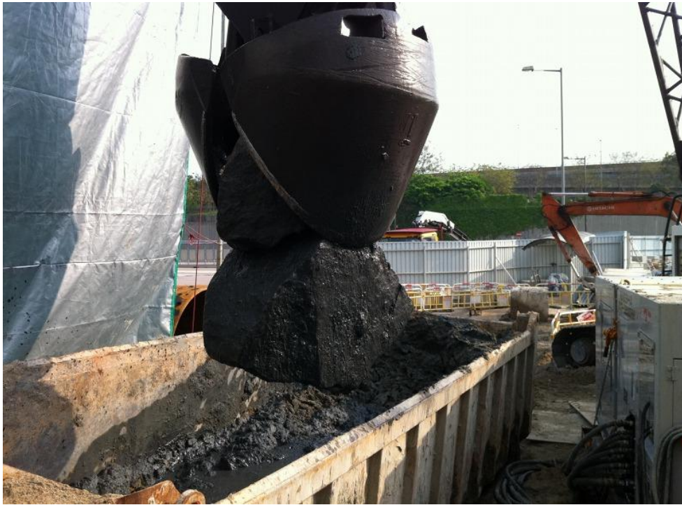
Boulder removal (転石撤去状況)
