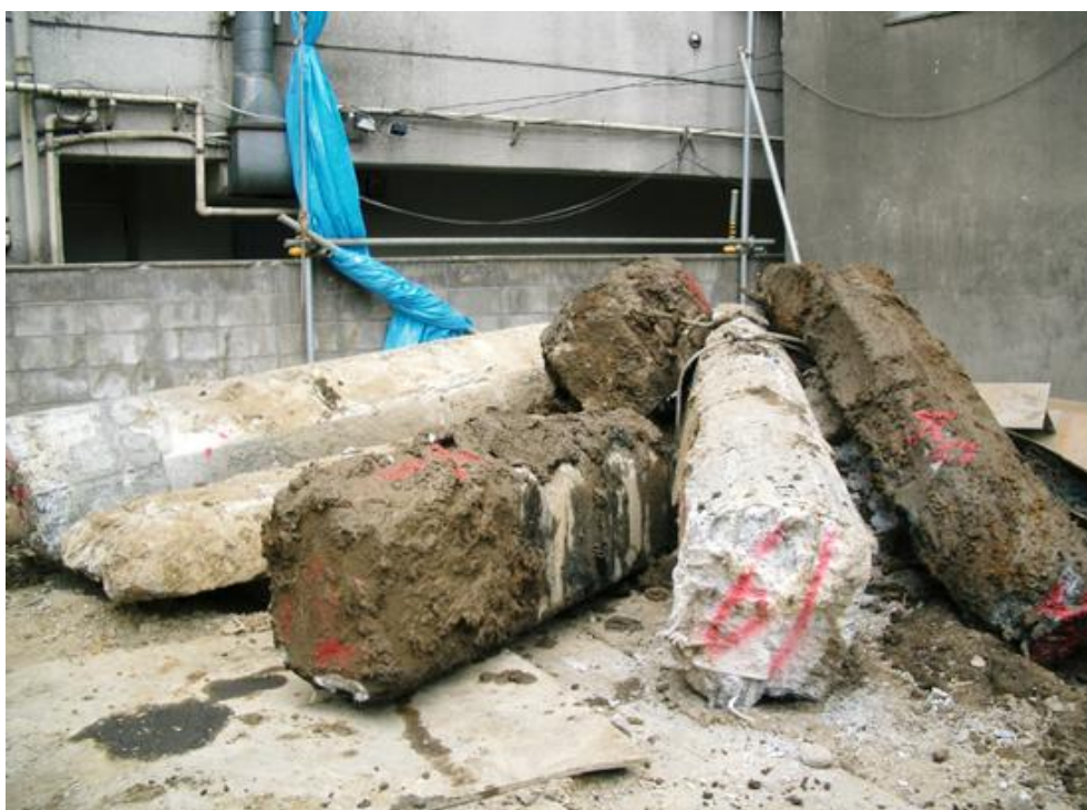
Underground obstacle removal situation (地中障害物撤去状況)
