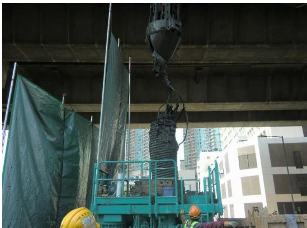
Removal of cast-in-place pile (場所打ち杭撤去状況)
