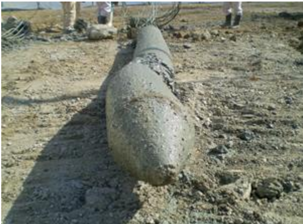
Underground obstacle removal situation (PC-pile) (地中障害物撤去状況 PC杭)
