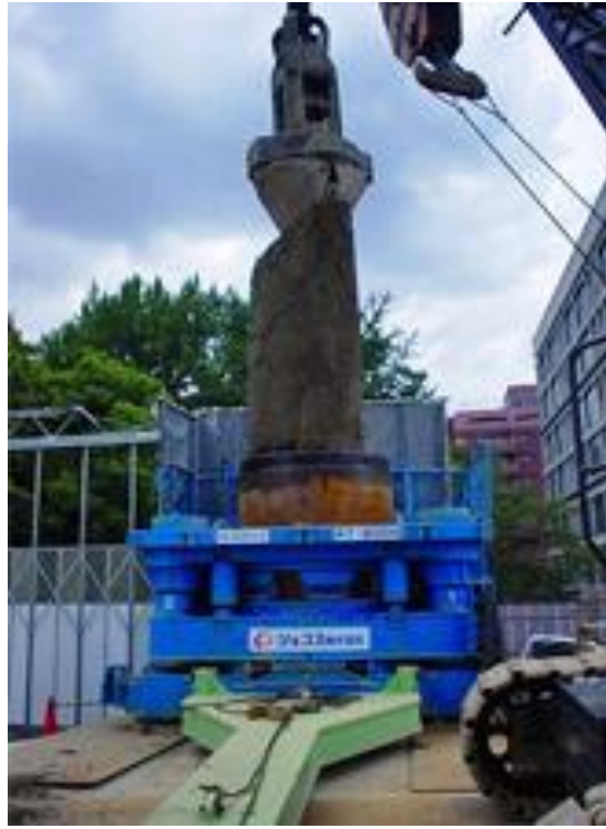
Removal of cast-in-place pile (場所打ち杭撤去状況)
